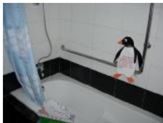
Safe Elderly; handrails in bath
